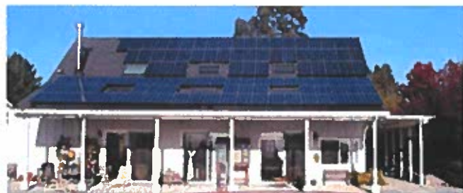
Two examples of roof arrays designs which detract from the integration with the roof.
