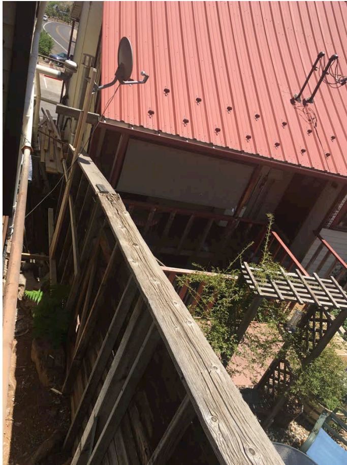
View from back of 538 School St., looking down trough toward Main St./89A
