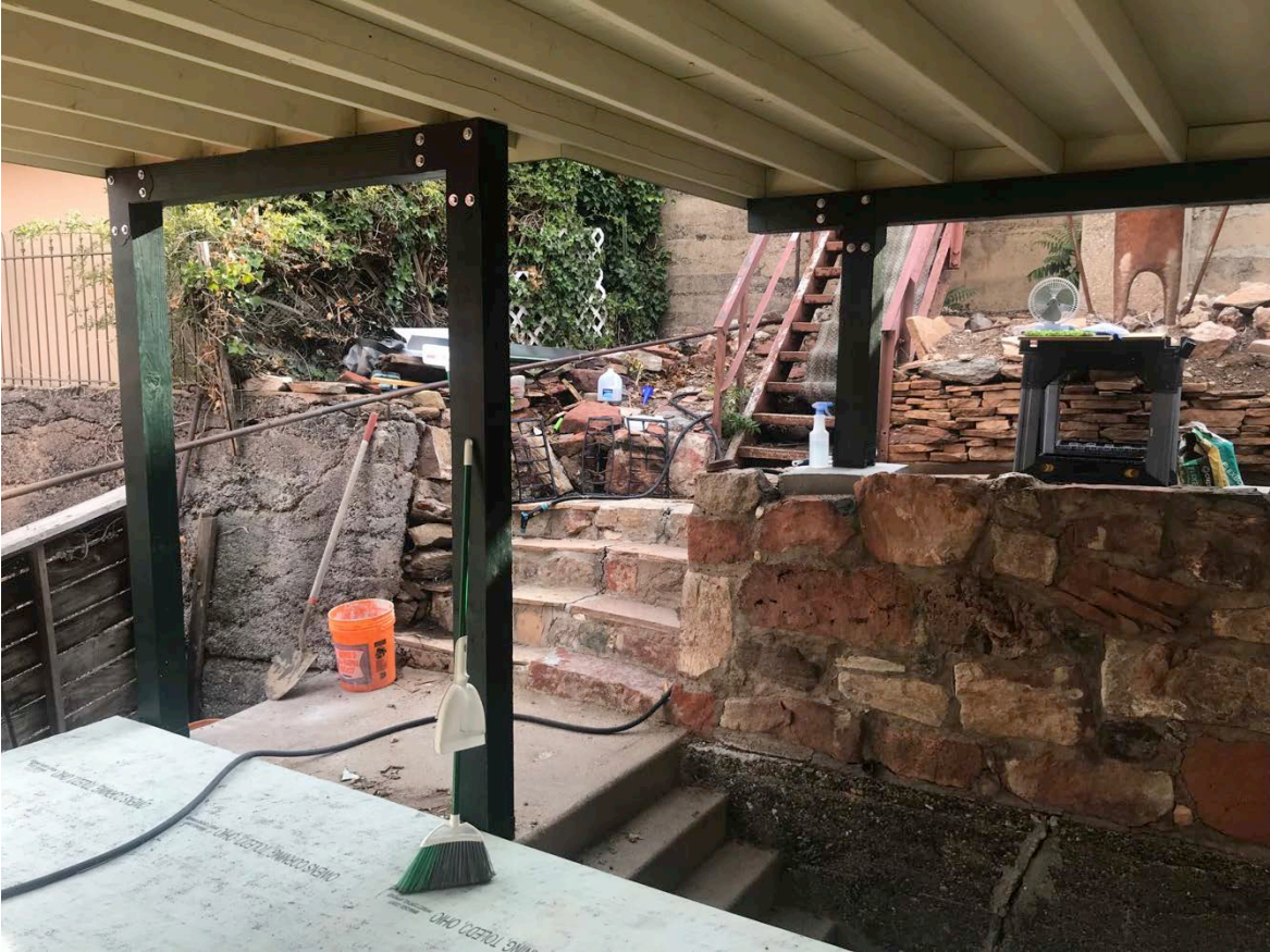
View from under porch roof looking toward dangerous steps, backyard and up to School Street.
