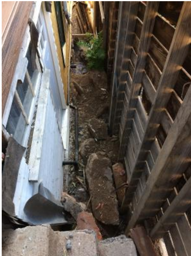
Close-up view from back of 538 School St., looking down trough toward Main St./89A
