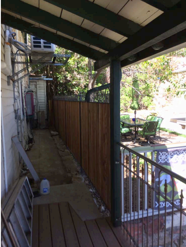
Vina Zona side of house. Walkway at 538 School St./539 Main St. from back deck to front steps. Vino Zona yard on right side behind screening fence we installed.
