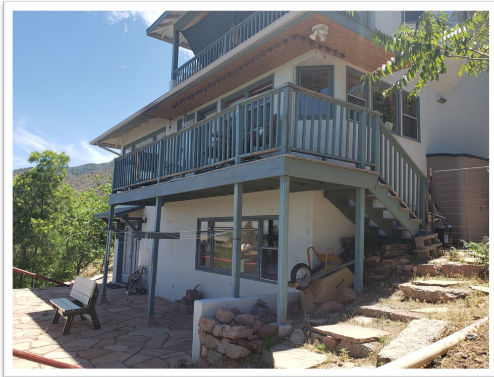
Existing deck that extends 5' from house
