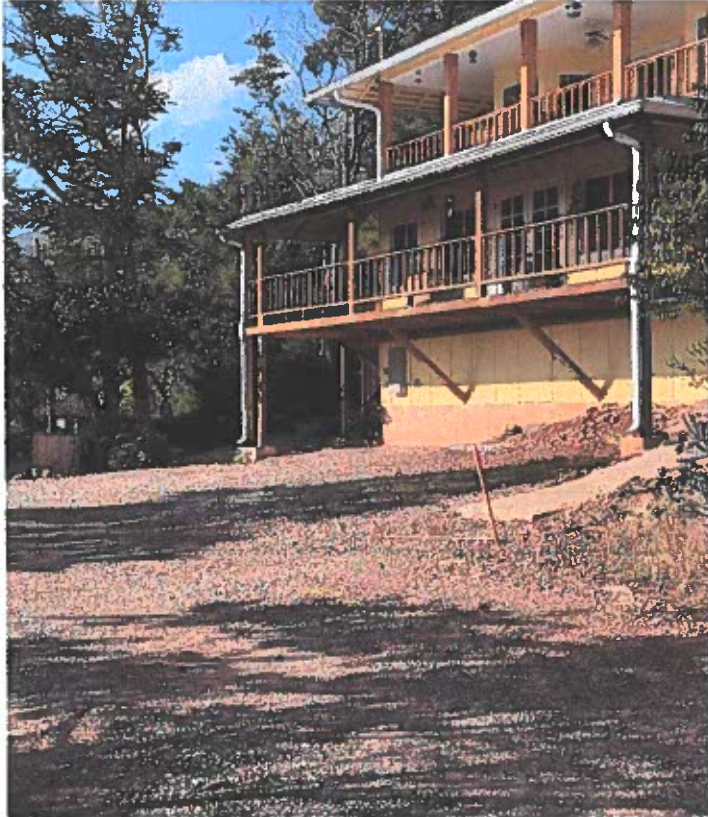
This is the Porchowski House with the survey marker showing the edge of the property. The house is set back less than 13' from the ROW
