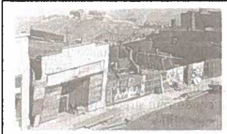
Men working on demolishing unstable buildings on Main Street, 1937 Figure 7. EXISTING structural damage to building on Main Street circa 1937 (Now SR 89A) (Jerome Historical Society)
