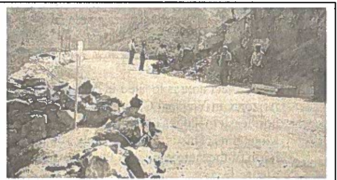
Figure 2. 1937 stone retaining wall construction (Clements 2003)
