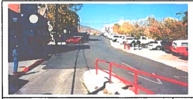
Figure 6. Present day Main Street, exhibiting missing buildings in landslide affected area
