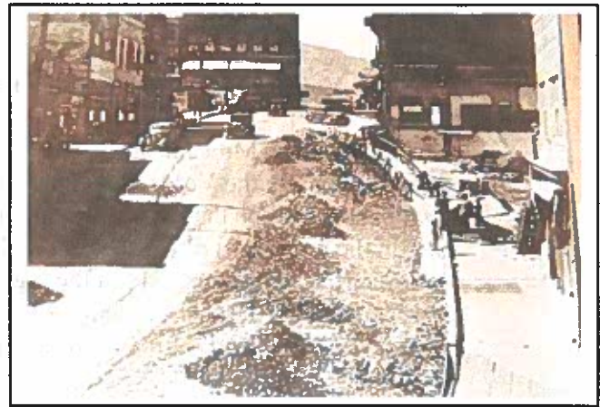
Figure 11. Fill and regrading of Main street was a common occurrence during the 1930's and 1940's
